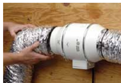
Connect the ducts.
